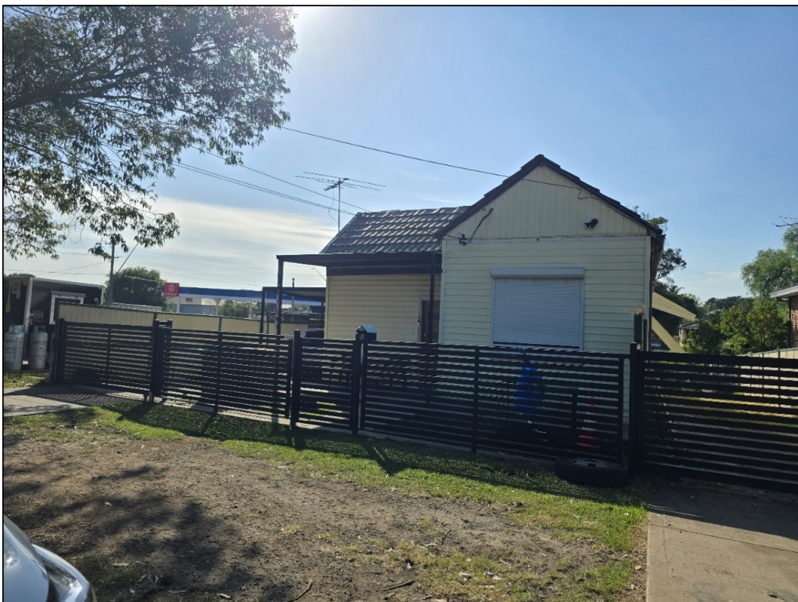
Figure 3 – Street view of subject site
